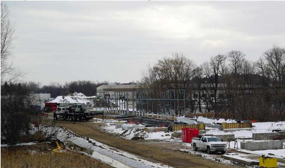
It is starting to look like a station. With most of the structural steel in place, the shape of the roof canopy and lantern features are clearly visible. (Looking south towards the Golden Triangle Station)
