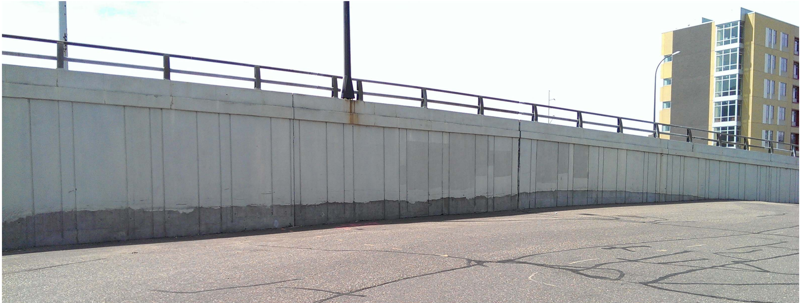
Existing Glenwood Ave. Corridor Wall Treatment – North Elevation View
