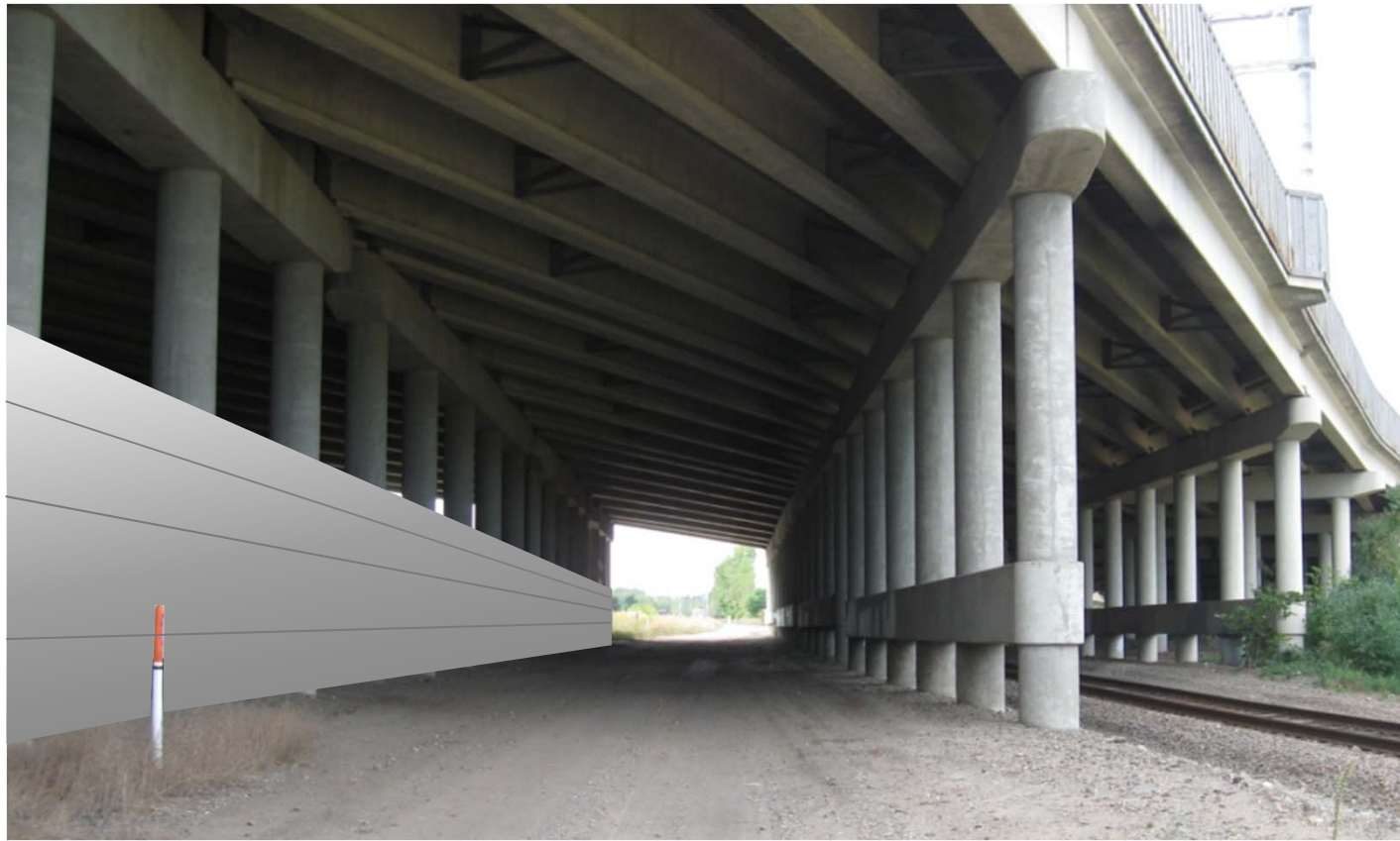
Extensive existing pier protection beneath I-394 with simulated crash protection walls.
