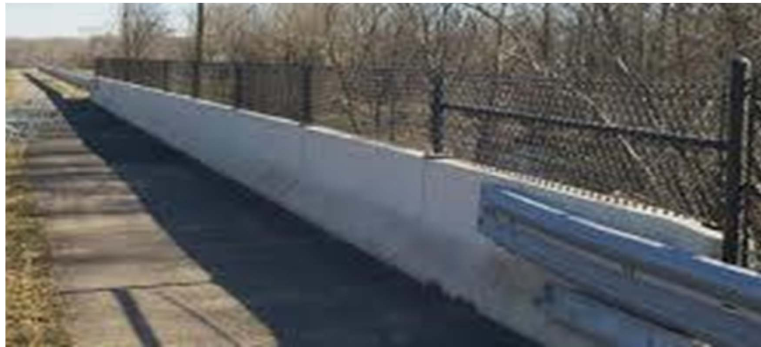
Example of safety fence on pedestrian bridge
