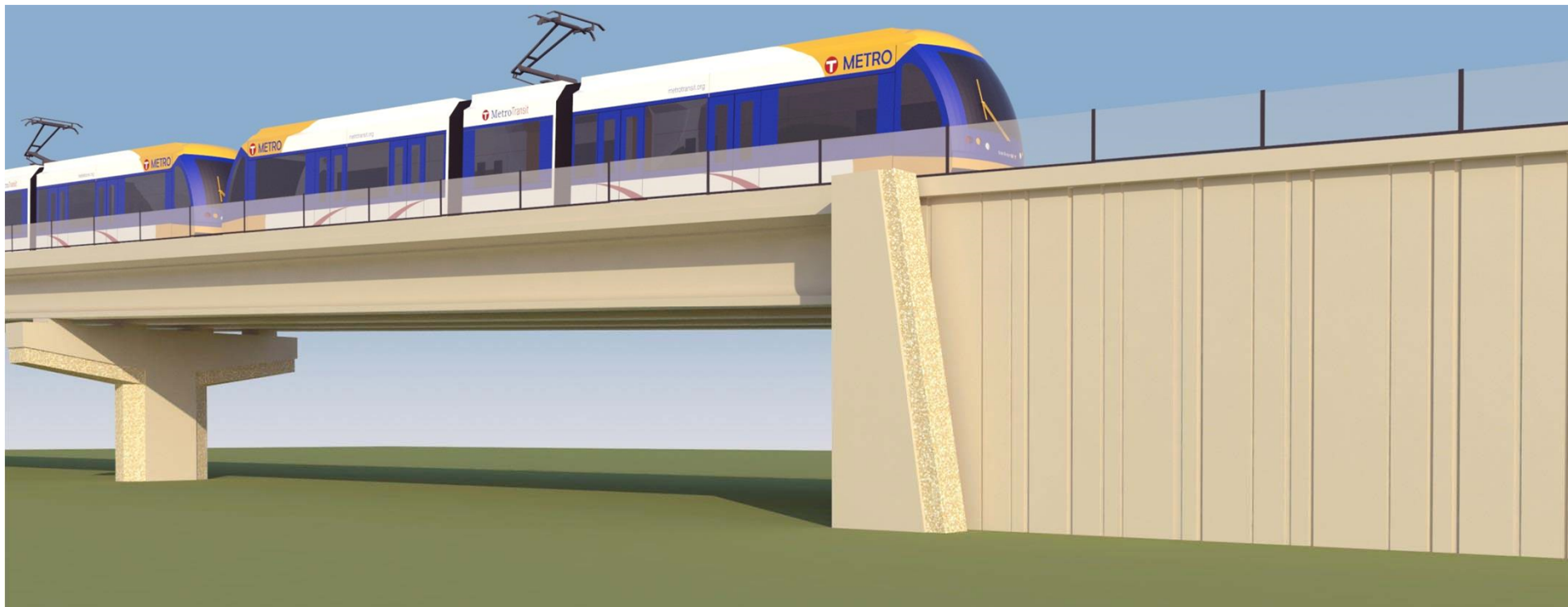
LRT bridge pier with base pilaster only
