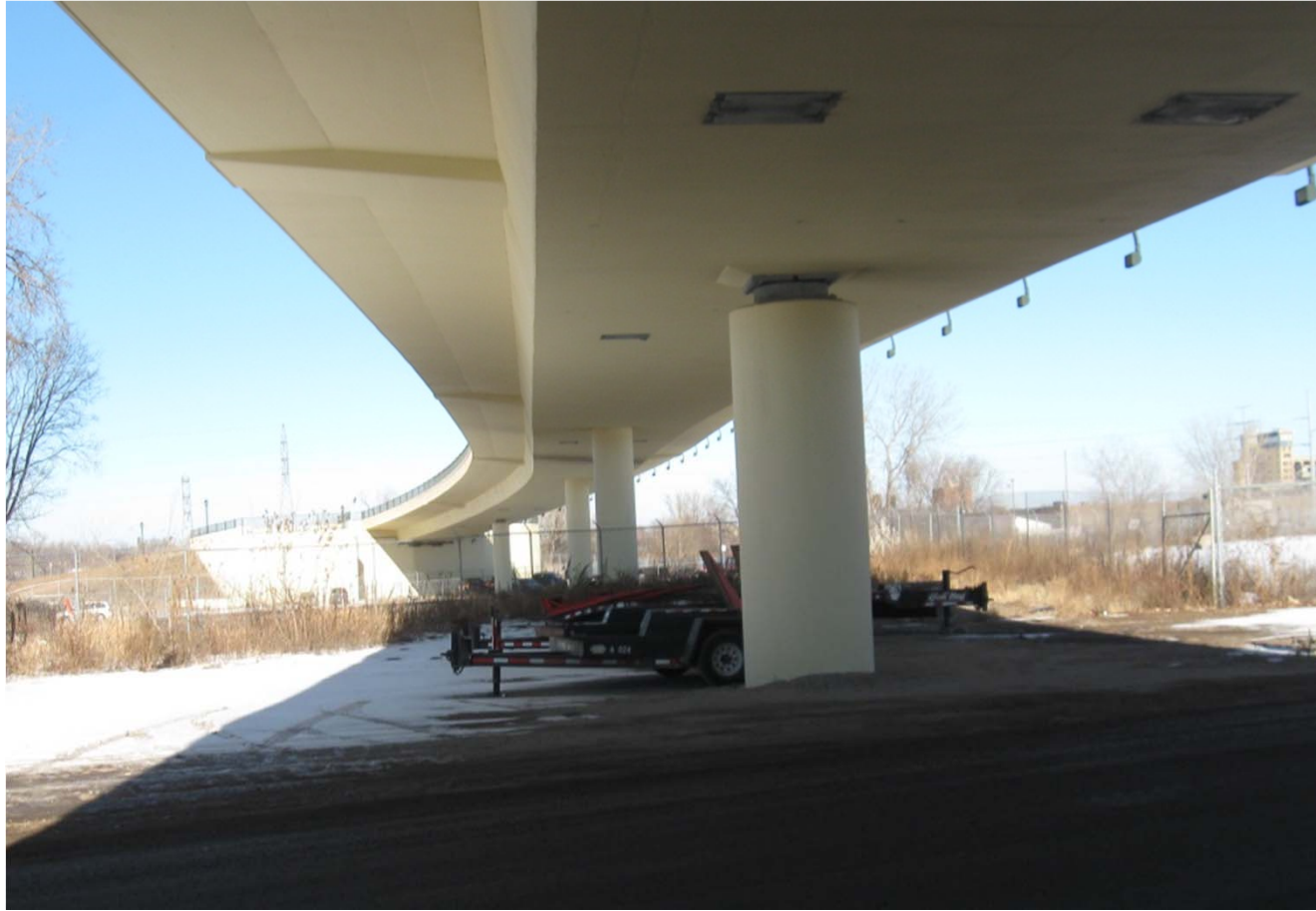
Existing Cylindrical Shaft Piers - Van White Memorial Blvd. Bridge
