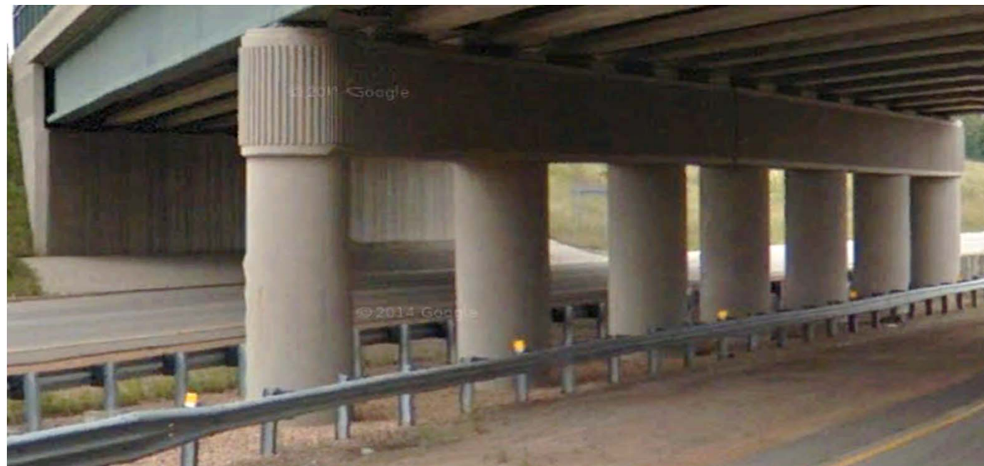
Example of Pier Cap Treatment
