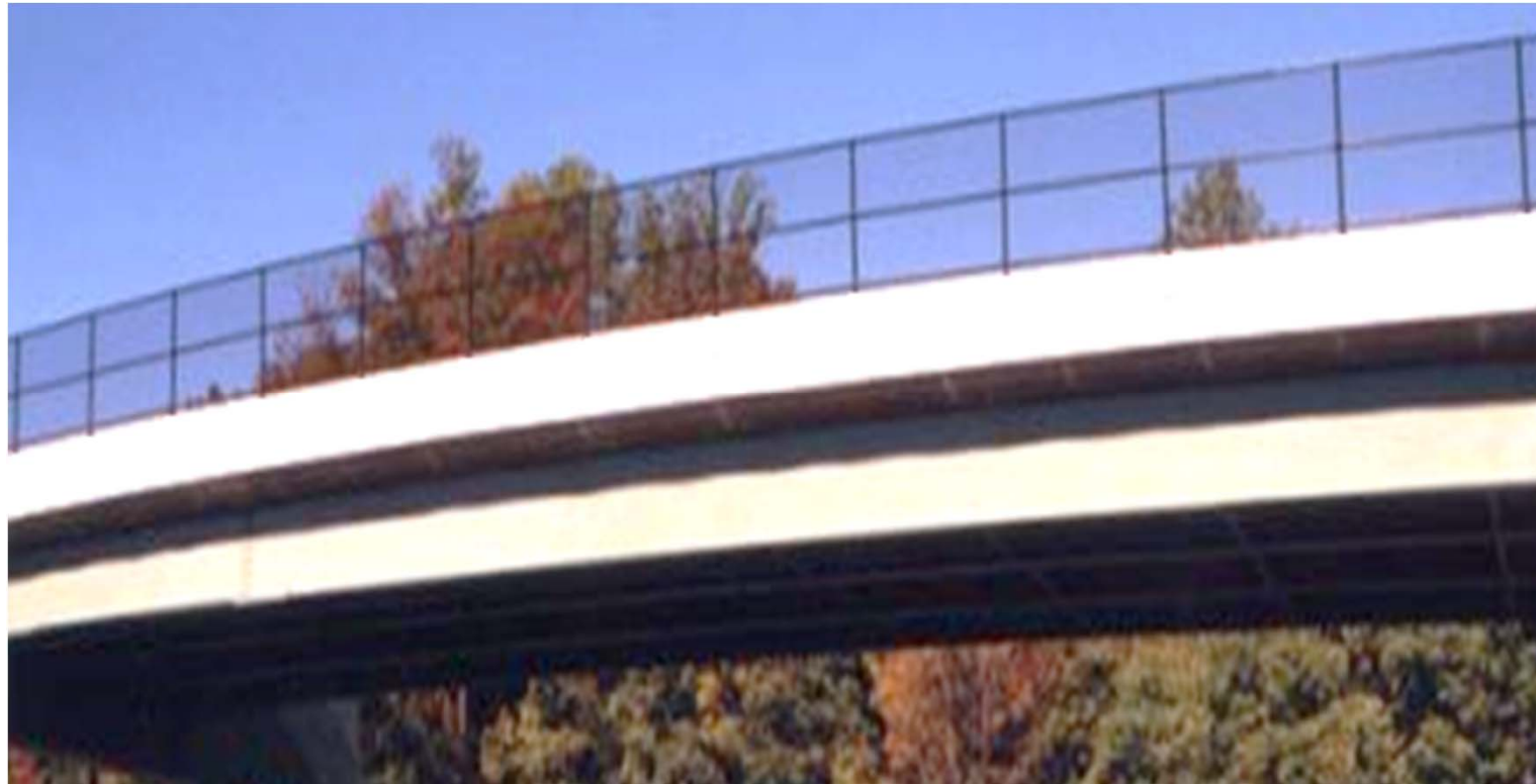
Example of Diamond mesh safety Rail on LRT bridge
