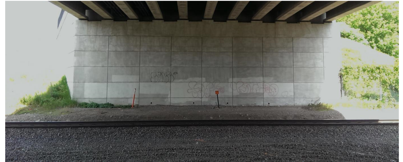
Existing Royalston Ave. - North Bridge abutment at Cedar Lake Trail
