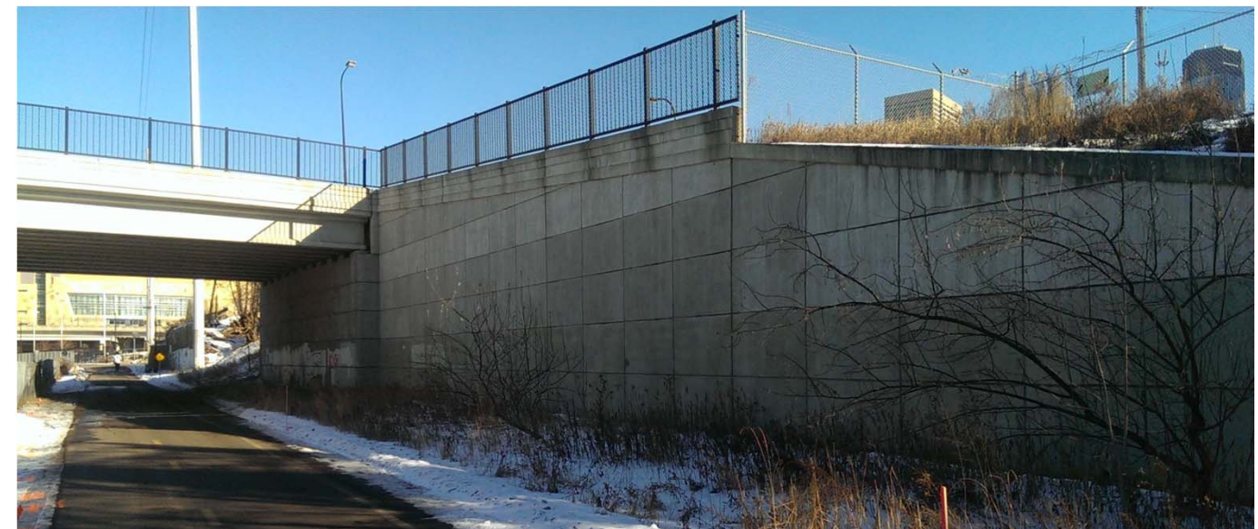
Existing Royalston Ave. - South Bridge abutment and retaining wall at Cedar Lake Trail
