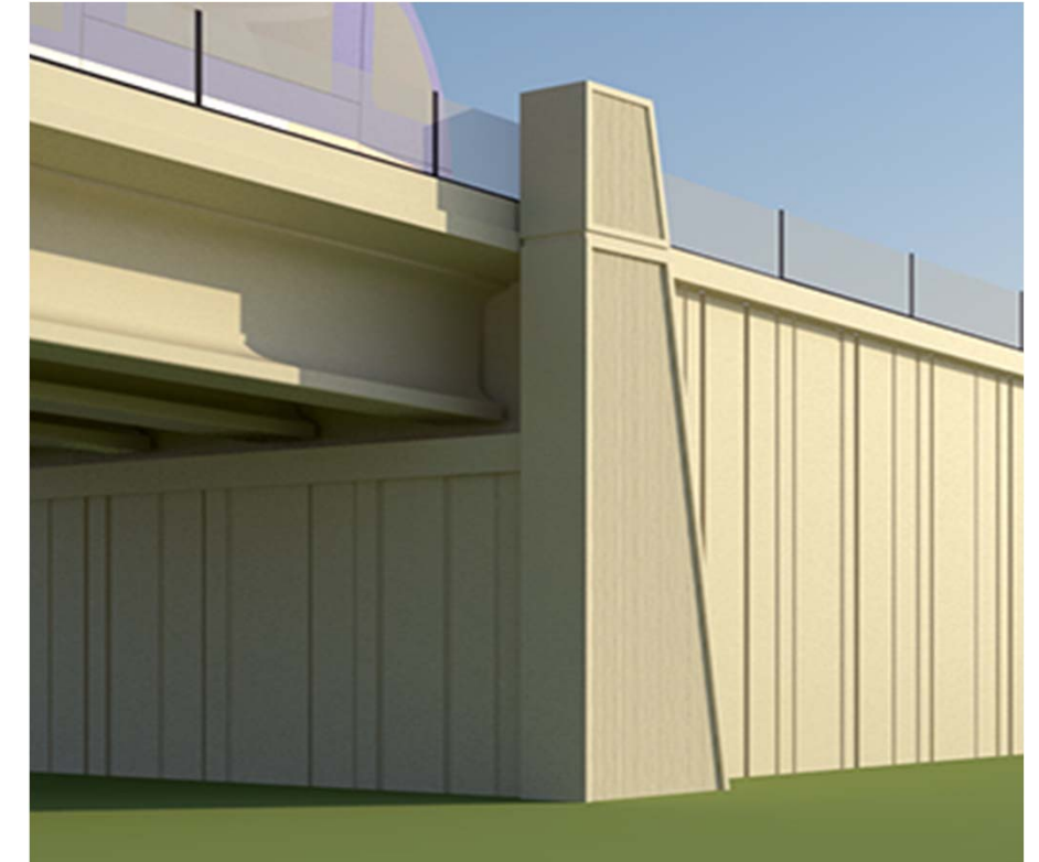
LRT bridge - abutment view
