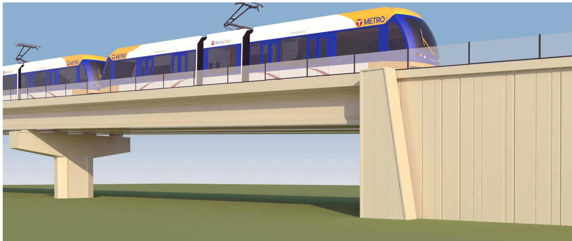
LRT bridge pier with base pilaster only
