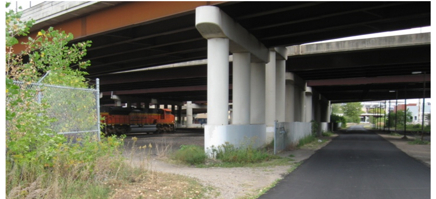
Extensive existing pier protection beneath I-94 with simulated crash protection walls.
