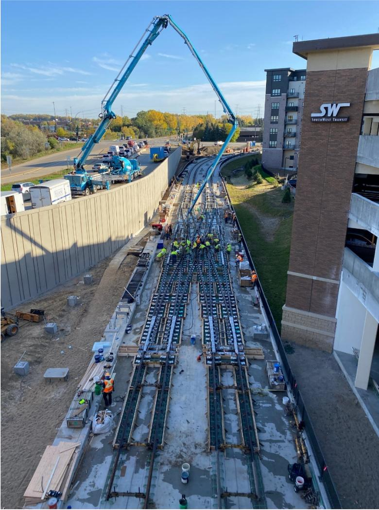
Crews work to install crossover tracks on the Prairie Center Drive Bridge as LRT enters the SouthWest Station. Crossover tracks allow light rail vehicles to move to the other track for maintenance or return trips.
