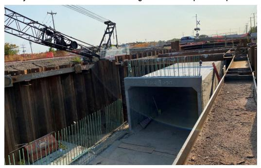
The Blake Road Regional Trail underpass is being constructed in two halves. With the west side of the tunnel structure complete, crews are building the east half. As pictured, the east half structure is now nearly complete, and crews can work to bury the underpass and complete finishing details.
