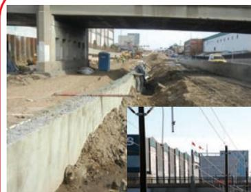
View of University Avenue near Cleveland Avenue looking east toward Prior Avenue. By fall of 2012, the roadway, guideway, embedded track, and landscaping has been constructed. Part of the systems work for this area was also completed by erecting the large center poles hanging the wires called the overhead catenary system.
