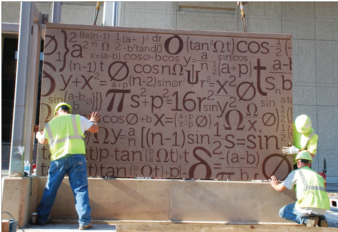
Workers installed artwork in mid-July at the East Bank Station.
