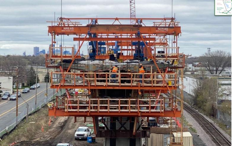
**Exterior Rebar and Form Work for Excelsior LRT Bridge, Hopkins**
