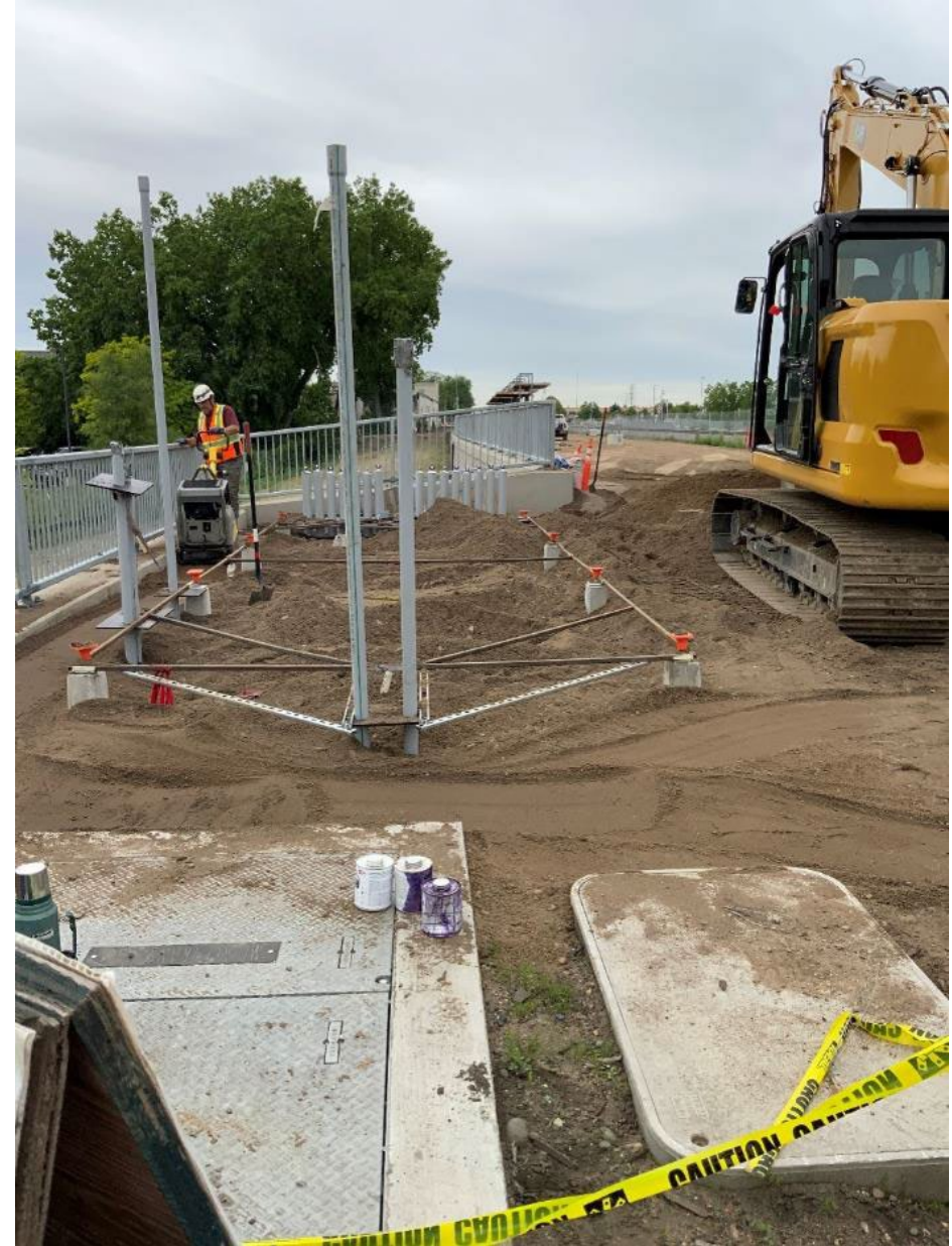
Wooddale Station Signal House Foundation Backfilling and Completion
