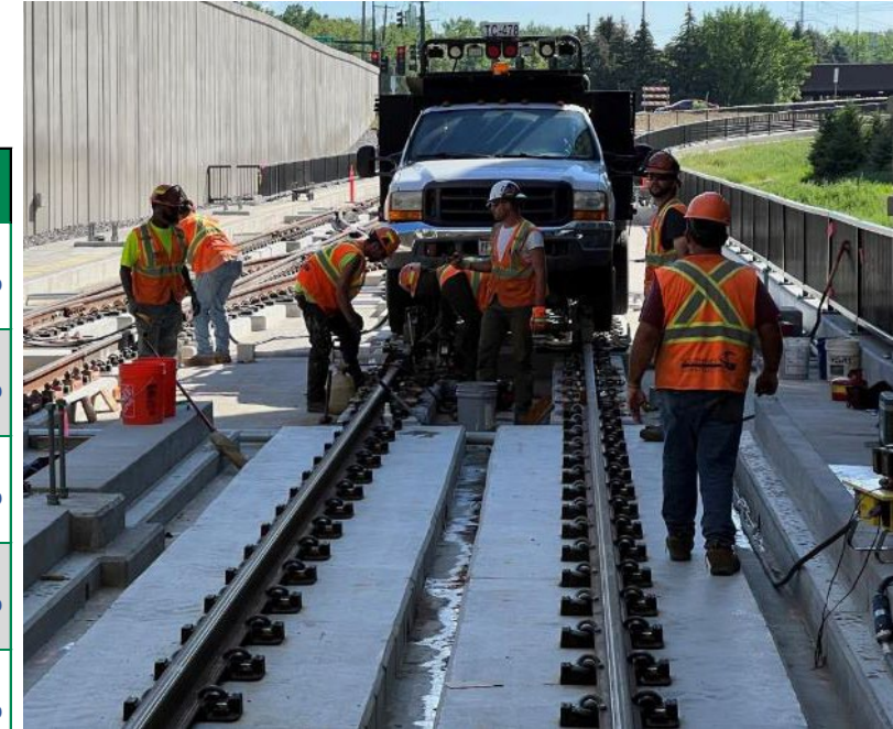
Track installation at SouthWest Station
