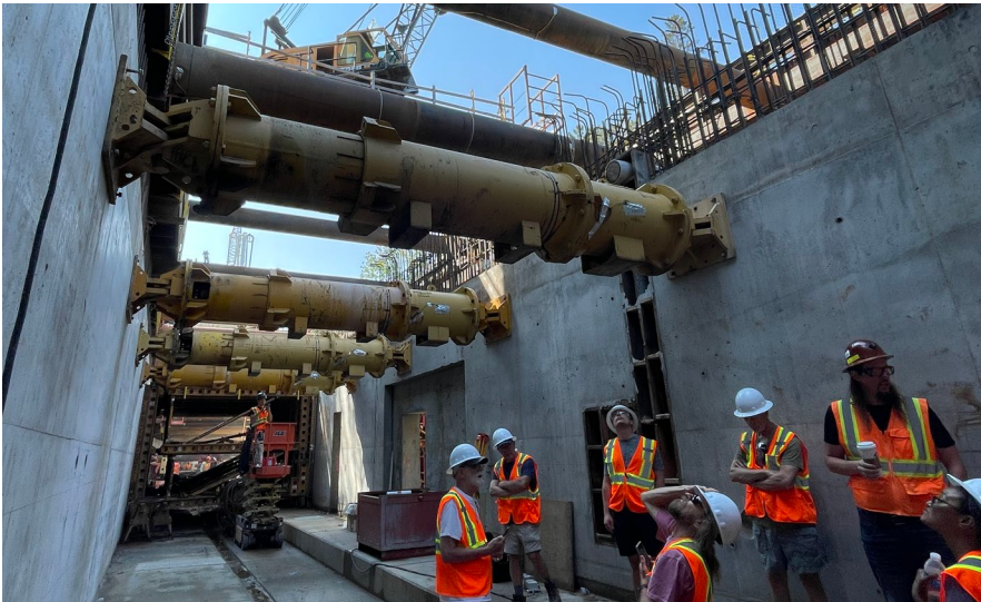
Kenilworth LRT Tunnel Tour, September 2024
