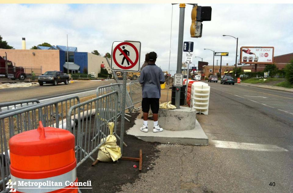
Action: Temp bus stop with ramp and protective railings, barriers and trash cans
