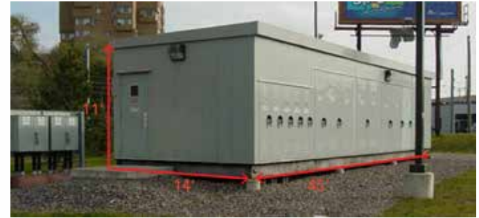
Traction power substation
