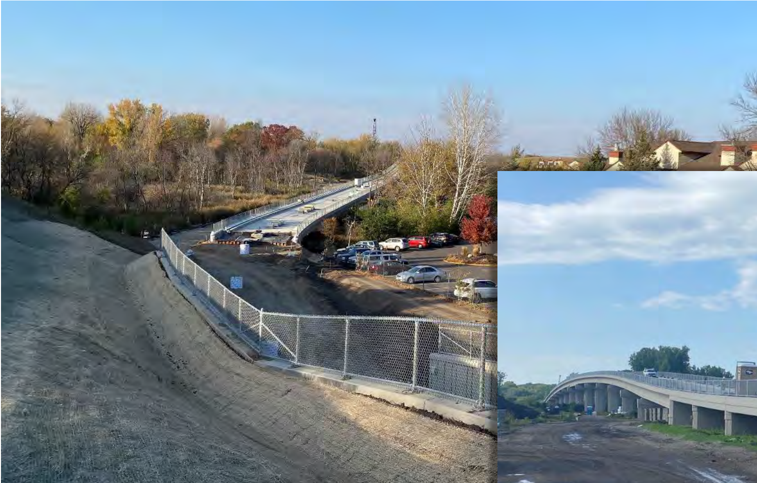
View to the North
